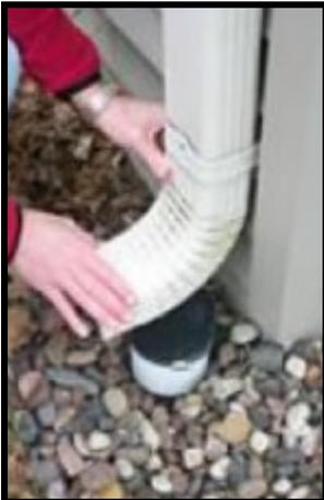
Attach the downspout pipe extension to carry water away from the house and foundation. You can use a hacksaw to cut the extension to the desired length. Be sure to insert the elbow into the extension to prevent leaks. Secure the elbow and extension with sheet metal screws. To prevent erosion where the water drains, you can place a splash pad at the end of the downspout extension.
